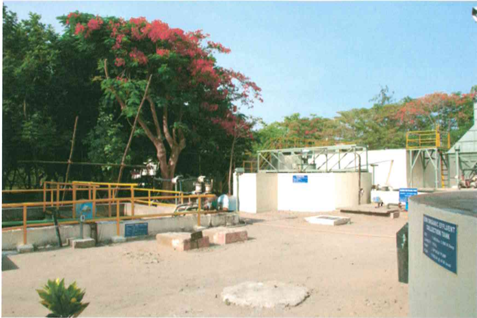
Greenery in ETP - around Chemical Rxn. Tank and Clarifier
