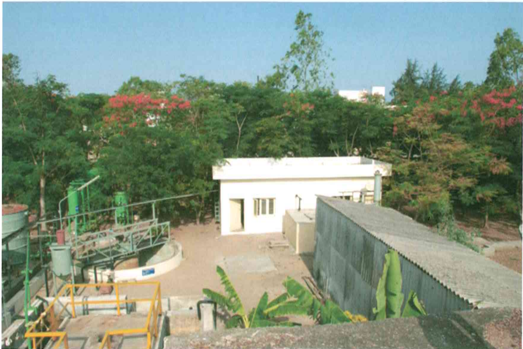
Greenery in ETP - rear side of RO plant
